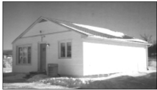
Figure 4. IRC Test House #1 with above-ground portion of basement visible
