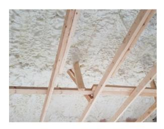
FOAM-LOK 450 is well-suited for new construction and retrofit applications in both residential and commercial buildings. FOAM-LOK 450 provides added value over traditional insulation, acting as an air, moisture and thermal barrier, and the product's excellent adhesion ensures that the insulation remains in place.
