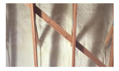
Keep your teams spraying without delays. HHuntsman Building Solutions ProSeal(TM) HFO is a high-performance medium density spray foam offering a very low global warming potential (GWP). This closed-cell product stands out with the following features:
