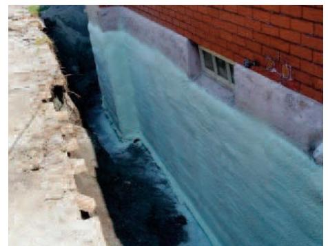
*Heatlok HFO is ideal for insulating old concrete or stone foundations from the exterior.*
