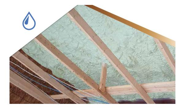
Classic LD-C-50 is a High Yield OC spray applied foam when installed following application guidelines, adheres tenaciously to framing members and substrates. Classic LD-C-50 is a low density, open celled, flexible, 100% waterblown polyurethane foam insulation. It is capable of being installed in wall cavities, roof assemblies (interior), attics, floor assemblies and ceiling assemblies.
