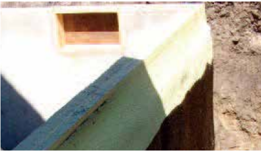
Bituminous coating applied directly over the foam.
