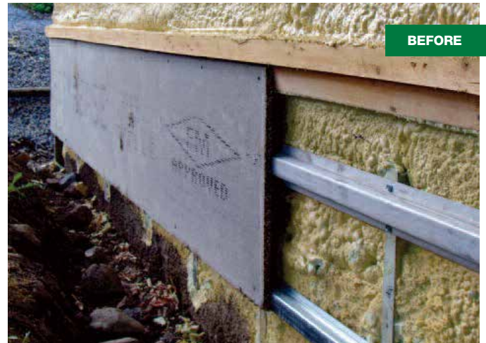
During application of spray foam and z-bars
