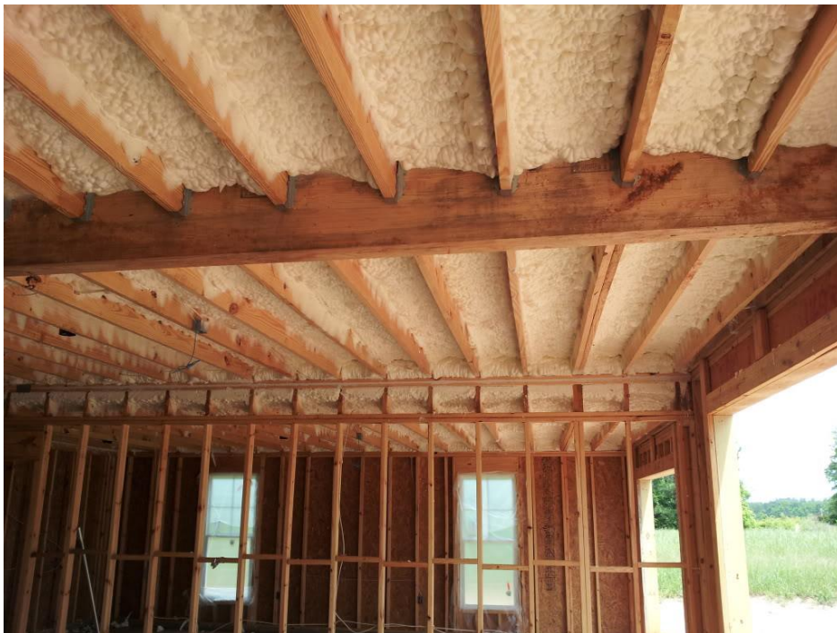
Figure 1. Example of application where the product may serve as a thermal barrier over MD spray urethane ceiling cavity insulation (and joists) (1) within the ceiling of wood-frame garages. (Photo shows spray foam still to be protected with the DC 315 thermal barrier.)
