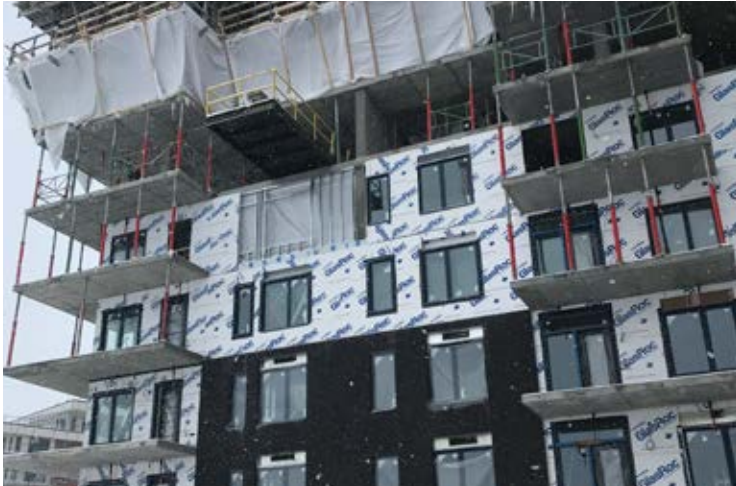
Example of productivity of the D-Max system. The cladding is installed from the ground floor to the third floor, the interior insulation is installed on levels 3 and 4 and the structure is poured on levels 6 and 7.
