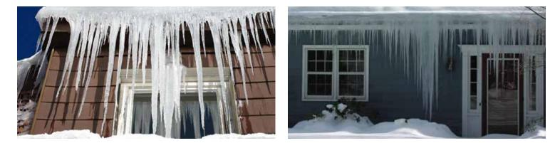
Roofs like these are frequently the source of problems, inside the structure and in the materials. The cause is often inadequate insulation and/or a discontinuity in the air barrier system.
