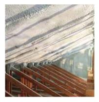
If you want a heated attic to use for storage, to install mechanical ventilation systems, or even to turn your attic into a living space, HEATLOK SOYA HFO can be sprayed directly onto the roof deck, with no venting. The soffits will have to be sealed and the attic will then be heated and completely sealed from the outside air. The same concept can be applied to a flat roof. Venting between HEATLOK SOYA HFO and the plywood sheathing is optional.
