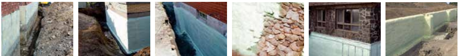
Heatlok Soya HFO is ideal for insulating old concrete or stone foundations from the exterior.
