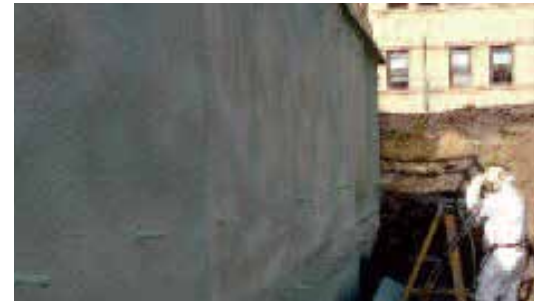
Drainage membrane that will be lifted in front of the foam as the soil is backfilled.
