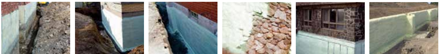
Heatlok Soya HP is ideal for insulating old concrete or stone foundations from the exterior.
