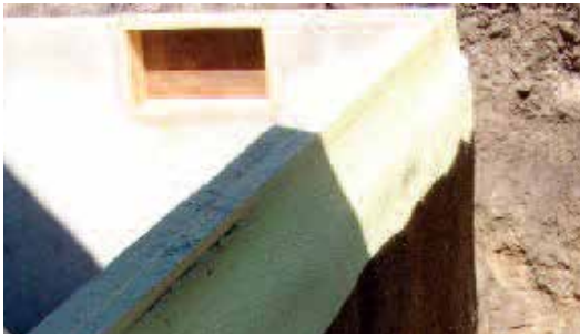
Bituminous coating applied directly over the foam.
