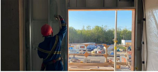
**4.** Spray Heatlok Soya HP according to the specified thickness.
