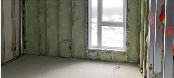
**5.** Installation of electrical systems. (This can be completed before or after the spray foam installation).
