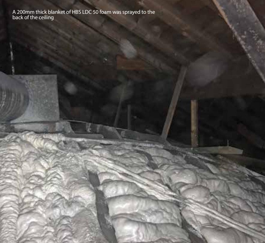
Access to the void between the roof and ceiling to the worship area was difficult for the Green Horizon, Icnene contractors
