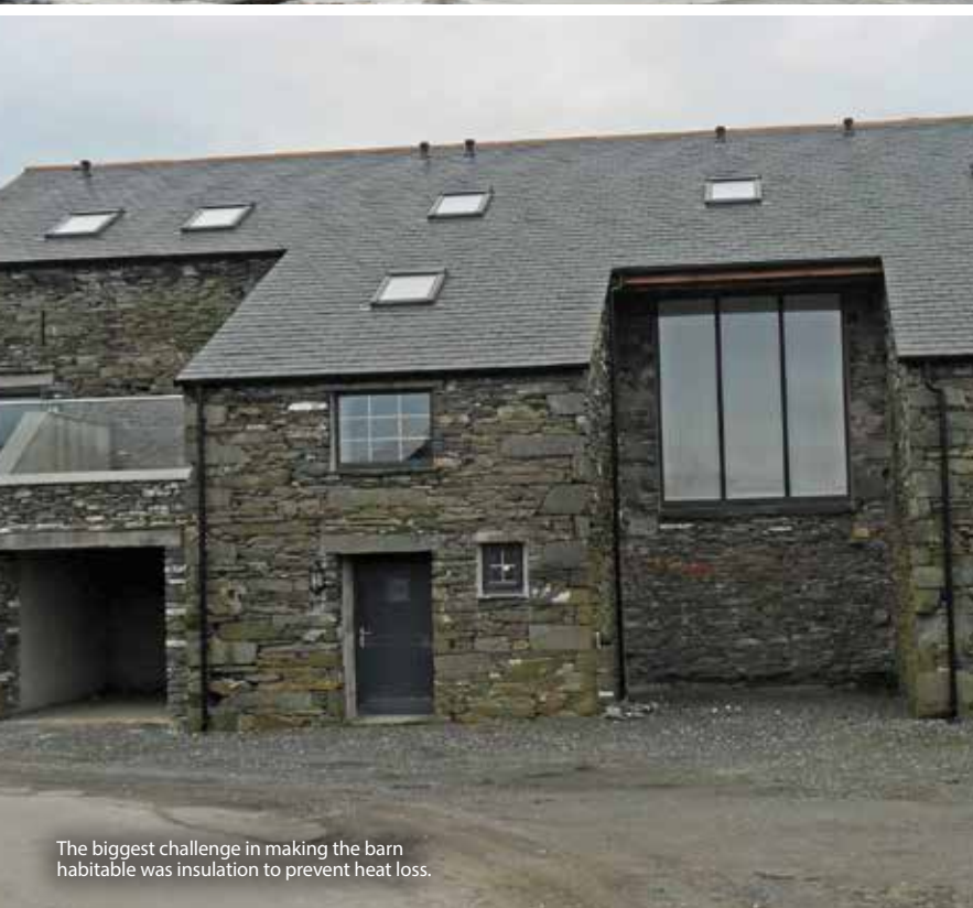
Two 2-bed cottages and one 3-bed house were created from the 19.0mx10.0m, three storey barn.
