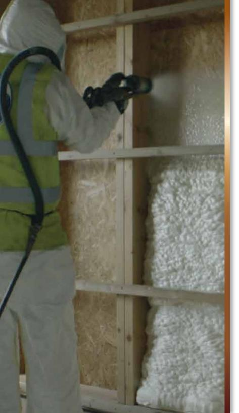
We asked Barry what it's like to work with spray foam from a professional perspective. "HBS spray foam insulation is really easy to apply for the technicians. It finishes really nicely and has the best thermal conductivity."
