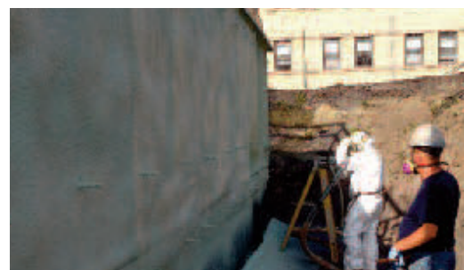
Drainage membrane that will be lifted in front of the foam as the soil is backfilled.
