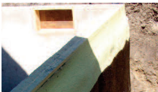
Bituminous coating applied directly over the foam.
