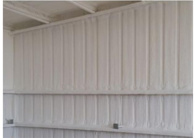
FOAM-LOK 2000 is a lightweight, durable, versatile insulation solution ensuring the highest performance in energy efficiency and energy cost savings. Closed-cell spray foam insulation systems, when properly installed, deliver energy savings of up to 40%.
