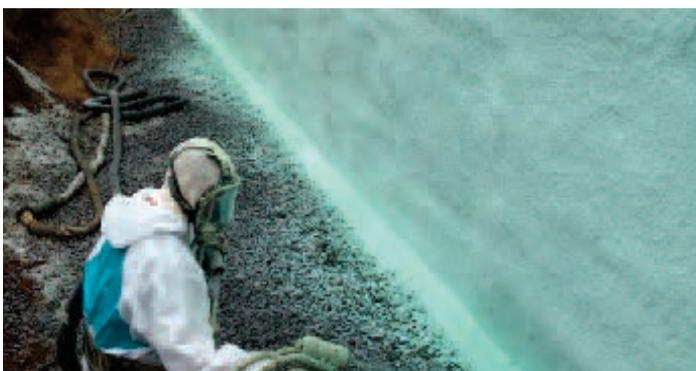
The ideal time and most effective way to insulate and waterproof the foundation is from the exterior while excavating an existing foundation and before backfilling a new foundation.
