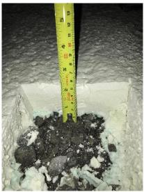
HL ccSPF is in 100% contact with its substrate making it very solid to walk on. Different thickness can be applied depending on the required R-value. 2" as demonstrated above is a common application.
