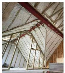
If you want a conditioned attic to use for storage, to install mechanical ventilation systems, or even to turn your attic into a living space, open-cell spray foam can be sprayed directly onto the roof deck, with no venting. The soffits and ridge vent will have to be sealed and the attic can then be conditioned and will be completely sealed from the outside air. The same concept can be applied to a flat roof. Venting between open-cell spray foam and the roof sheathing is optional.
