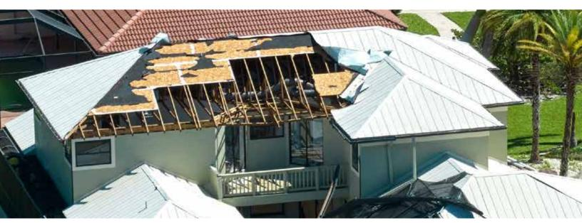
By sealing an attic with spray foam insulation, wind uplift damage can be reduced or eliminated altogether during severe weather.
