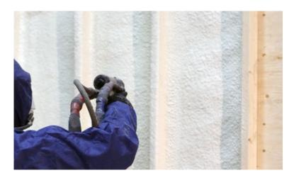
New advanced closed-cell, medium-density spray foam insulation. Huntsman Building Solutions ProSeal® sets a new benchmark in sprayability and performance. ProSeal offers a higher R-value and improved yield to meet today's strict building code requirements, making it ideal for residential applications. This low VOC spray foam insulation product allows for a higher initial pass of three inches to achieve R-21 as well as a Class II Vapor Retarder in one pass.
