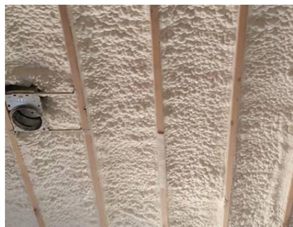
FOAM-LOK 500 is an open-cell spray foam insulation technology that is installed in interior spaces with no ignition barrier required.
