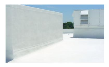
Thermo-Sil™ is a silicone elastomeric high-solids roof coating designed to provide reflectivity and renewability in a protective wear surface. It is a moisture cured roof coating designed to provide long-lasting performance in the most rigorous climates.
