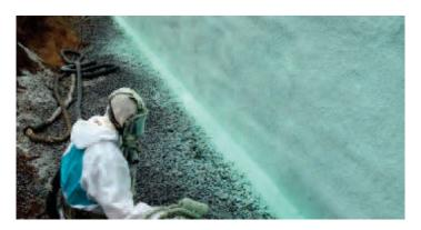
The ideal time and most effective way to insulate and waterproof the foundation is from the exterior while excavating an existing foundation and before backfilling a new foundation.
